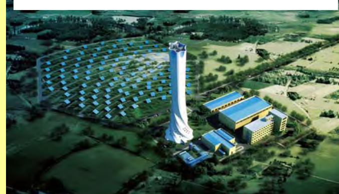
MW-level Tower-Type Plant in Beijing
